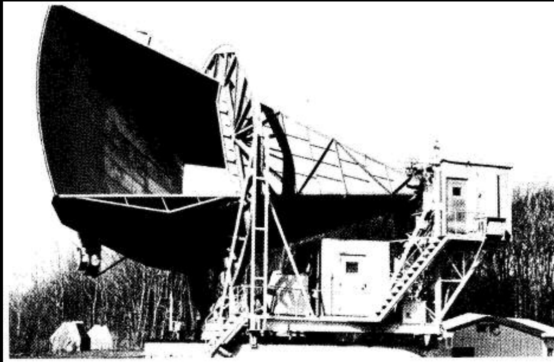
20-foot horn-reflector used by Penzias & Wilson
